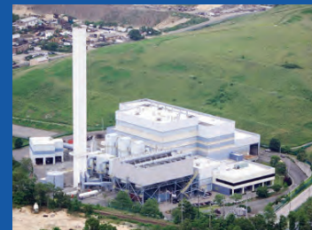
Covanta Huntington 99 Town Line Road East Northport, NY 11731
