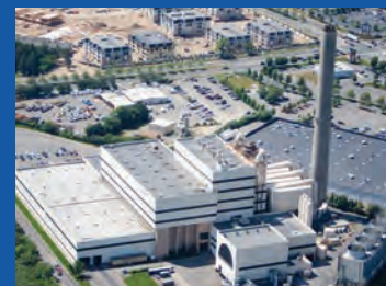
Covanta Hempstead 600 Merchants Concourse Westbury, NY 11590
